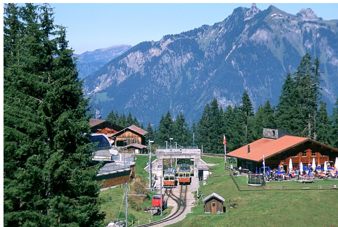
The BLM's only passing siding is at Winteregg, midway along the 2.6-mile-long tramway between Grutschalp and Murren.
